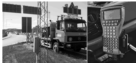
Fig. 1. Road inspectors taking care of a defective road sign (left). The current reporting-system used by the road inspectors (right).
